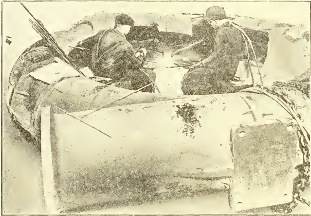
FIG. 158.—Building Up Worn Parts of Large Pump.
